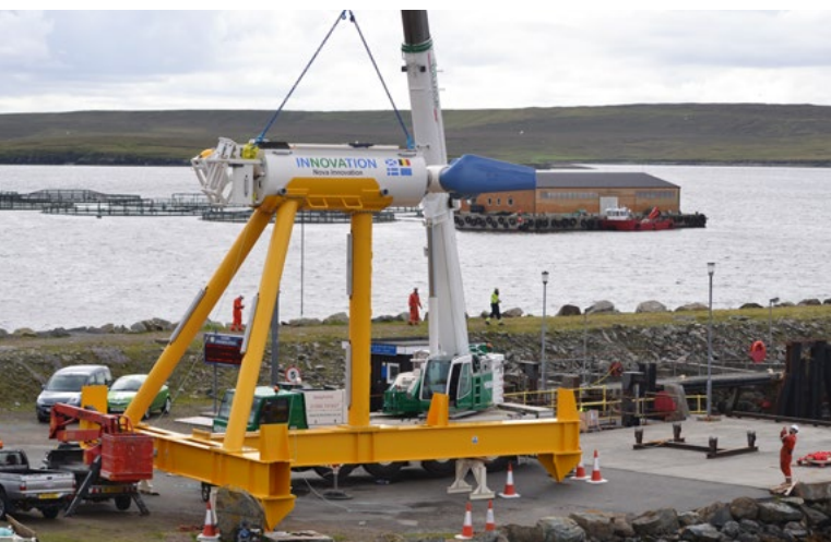
Nova Innovation M100 during assembly in Shetland Islands, Bluemull sound, UK Courtesy: Nova Innovation
