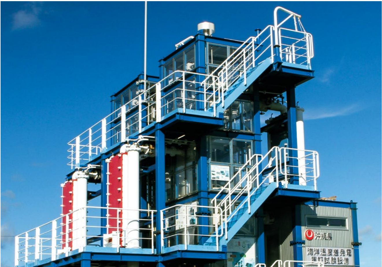
Okinawa Prefecture Deep Sea Water OTEC Demonstration, Kume Island, Japan Courtesy: Okinawa Prefecture
