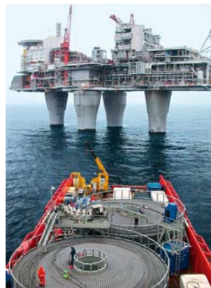
Troll-A oil platform in the North Sea and cable laying ship (ABB)
