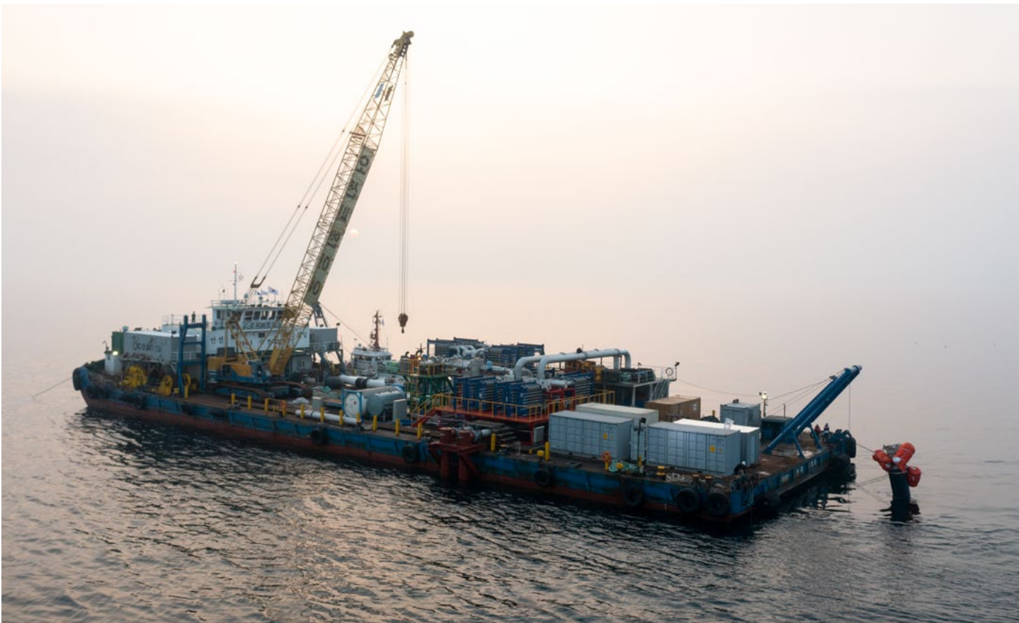
1MW OTEC Riser Installation at Pohang (Courtesy: KRISO)
